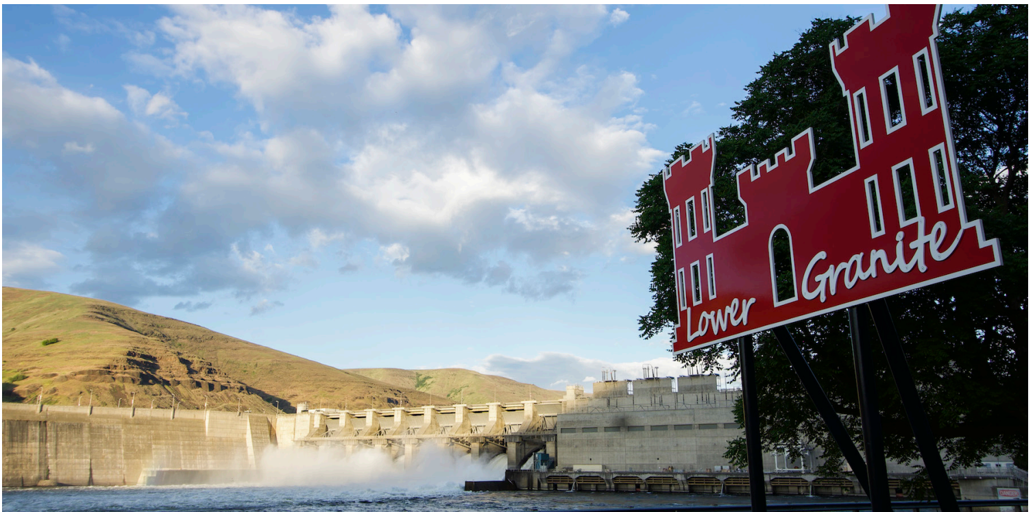
Lower Granite, one of the four Lower Snake River Dams. Despite significant investments to improve juvenile fish passage at these dams, salmon continue to spiral towards extinction.
