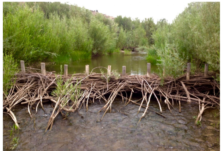
Figure 5: Beaver Dam Analag (BDA) in Bridge Creek. Photo courtesy of Utah State University.
