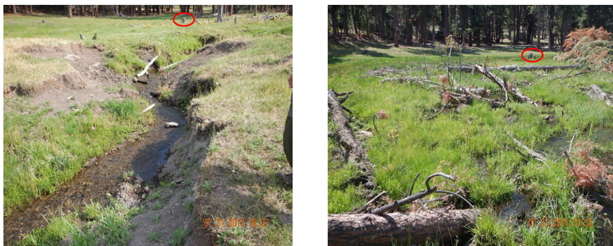
Figure 2: Restoration of a wet meadow in Eastern Oregon. Left: pre-restoration (July 2013); Right: one-year post-restoration. Red oval indicates the same tree stump, as a point of reference. Photo credits: Paul Powers.
