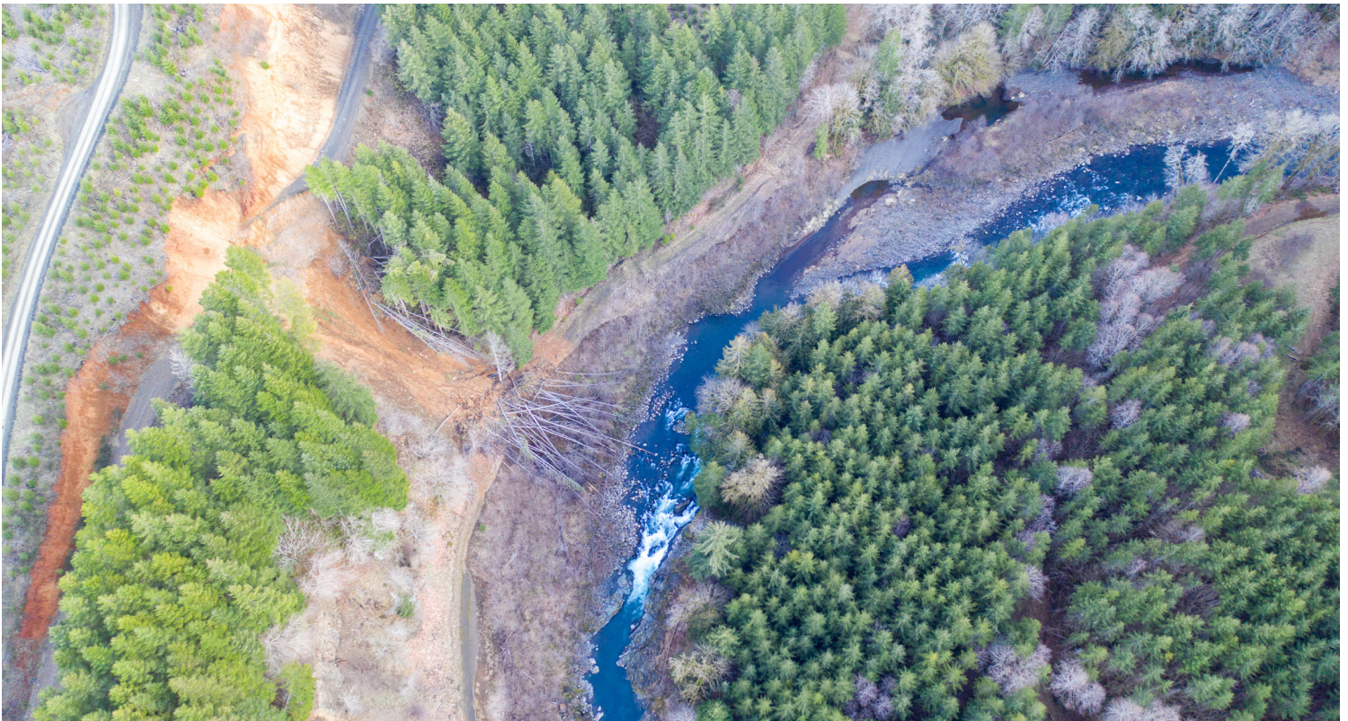
A recent landslide at the proposed dam site.
