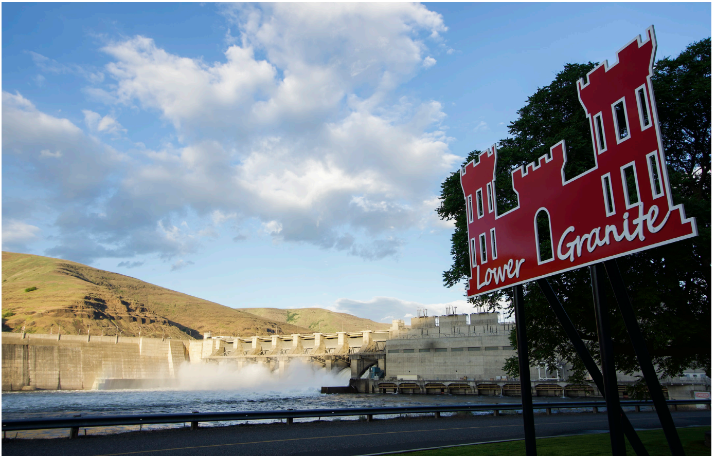
Lower Granite, one of the four Lower Snake River Dams. Despite significant investments to improve juvenile fish passage at these dams, salmon continue to spiral towards extinction.
