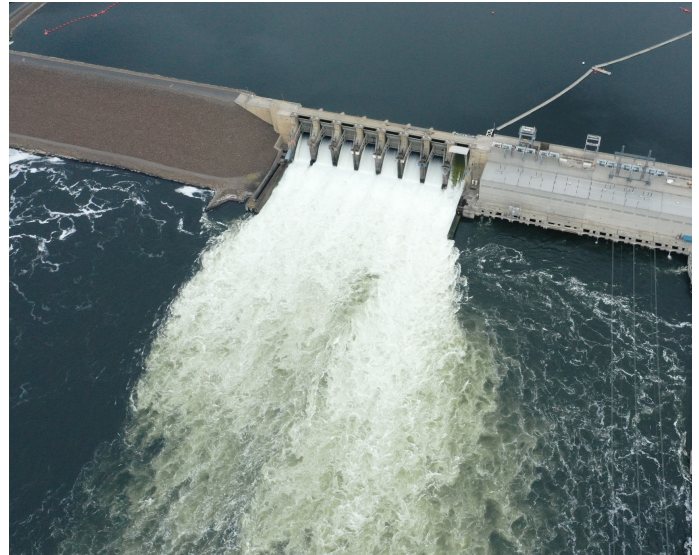
Little Goose Dam on the Snake River.
