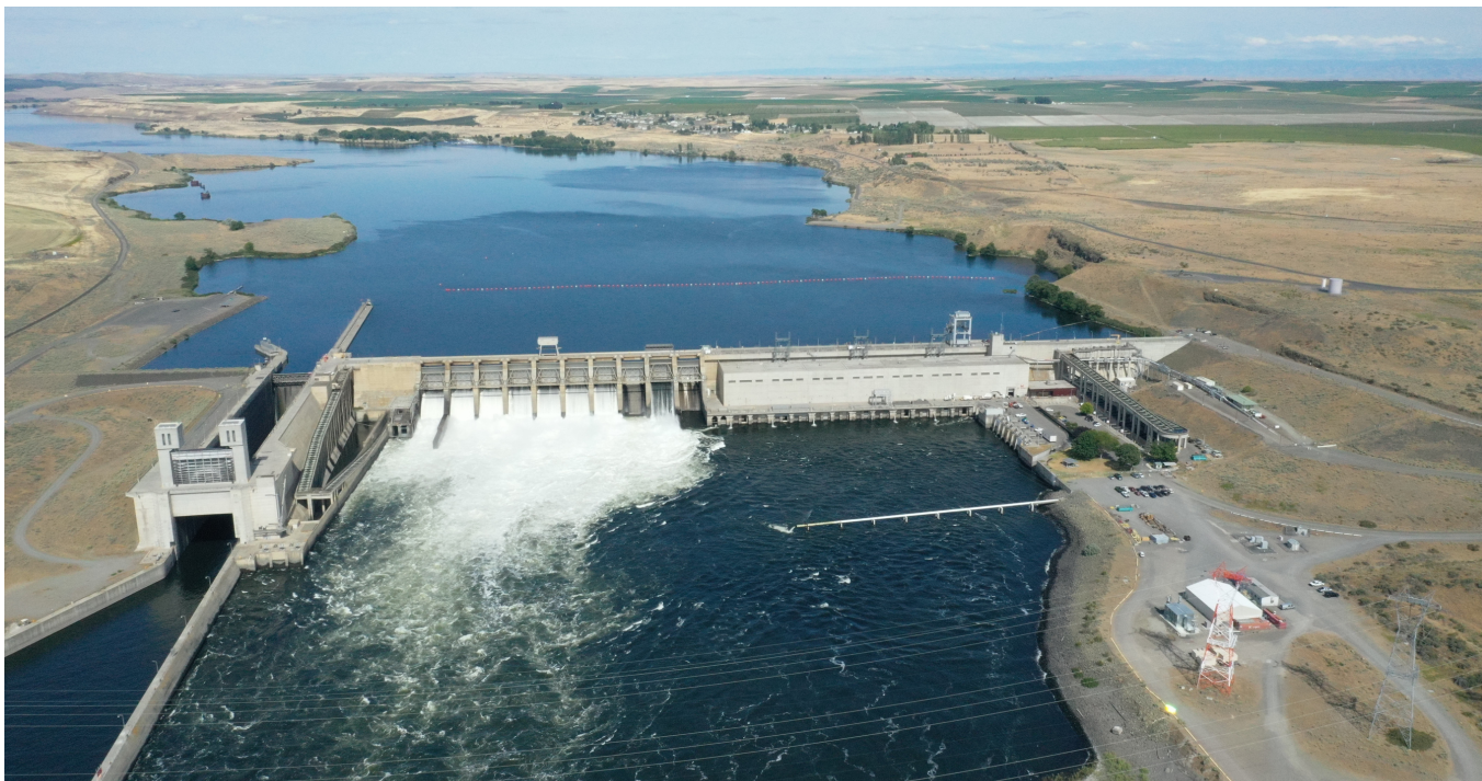
Ice Harbor Dam on the Snake River.
